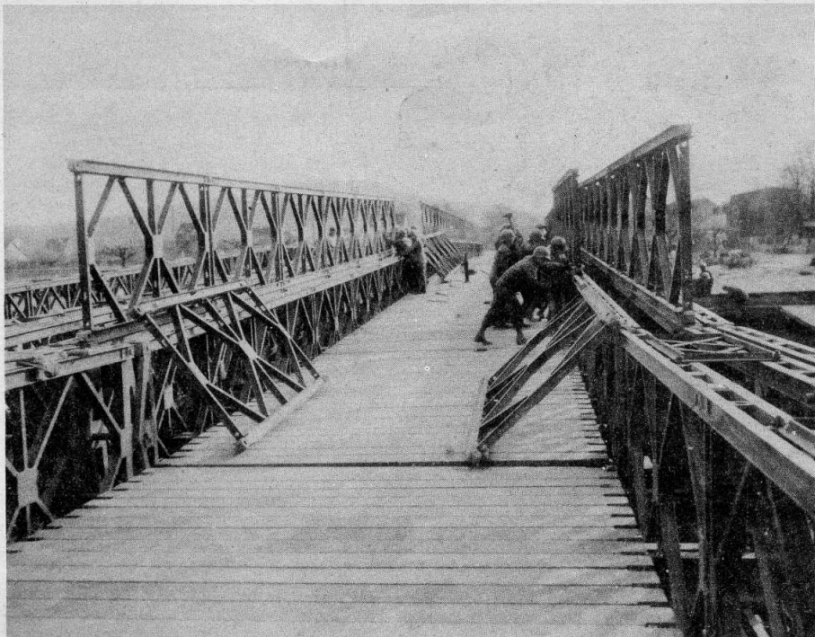
PLACING THE SECOND STORY ON THE CLASS 70 CARRIAGEWAY
